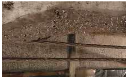
3. Coated beam and rebar
