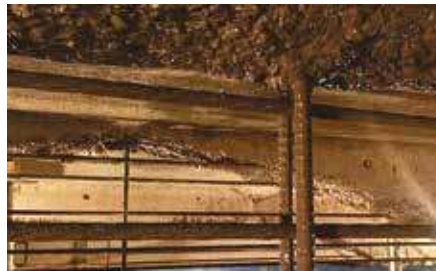
2. Coated beam and rebar
